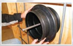
2. Attach INFINITY® wall sleeve to locator cap.
