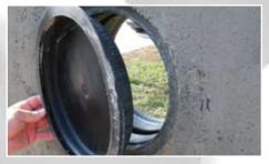
6. After concrete is cured, pry off the locator caps with a pry bar.
