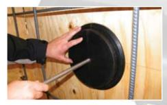
Extend (threaded rod\*) through form and first locator cap and (threaded nut\*) on the back side of form.
