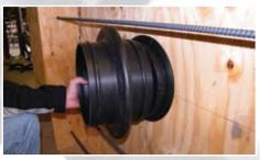
3. Cut the INFINITY® sleeve ¼" longer than the wall thickness. Insert the INFINITY® sleeve over the locator cap.
