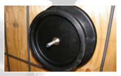
3. Slide second locator cap through (threaded rod\*), use fender washer and fasten nut until locator caps and sleeve is locked in place. Check to make sure sleeve is square to form.
