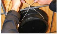
5. Attach the INFINITY® sleeve to the rebar using wire.
