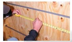
Using a tape measure, pull measurements from the horizontal and vertical positions to locate the center of the INFINITY® sleeve.
